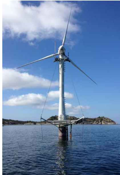
SWAY's one-fifth scale prototype demonstration wind energy system installed off the coast of Bergen, Norway. Photo by Eric Nelson, NREL/PIX 21966
